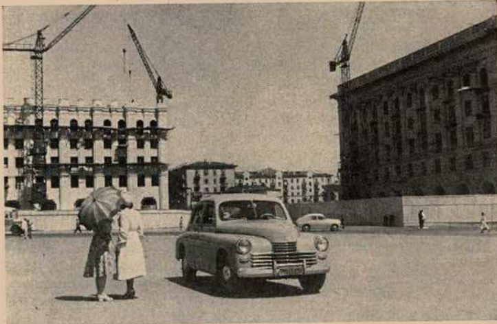
HUGE CRANES are left on the site until a building is completed—which may take years. Much of this time they are idle.
