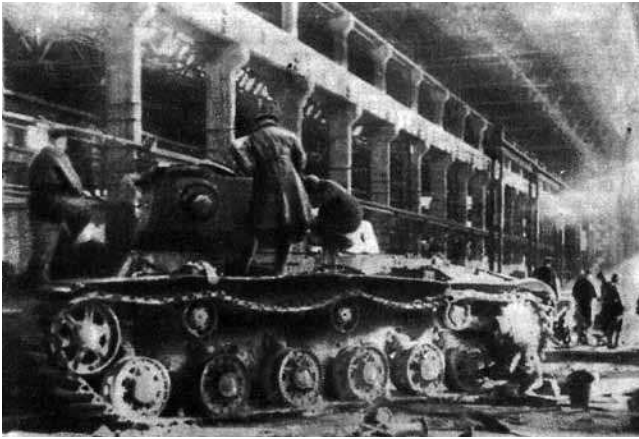
Figure 10. Soviet tank repair in the middle of battle, Stalingrad Tractor Plant. August 1942. Vokrug Sveta , no. 1 (January 1983).
