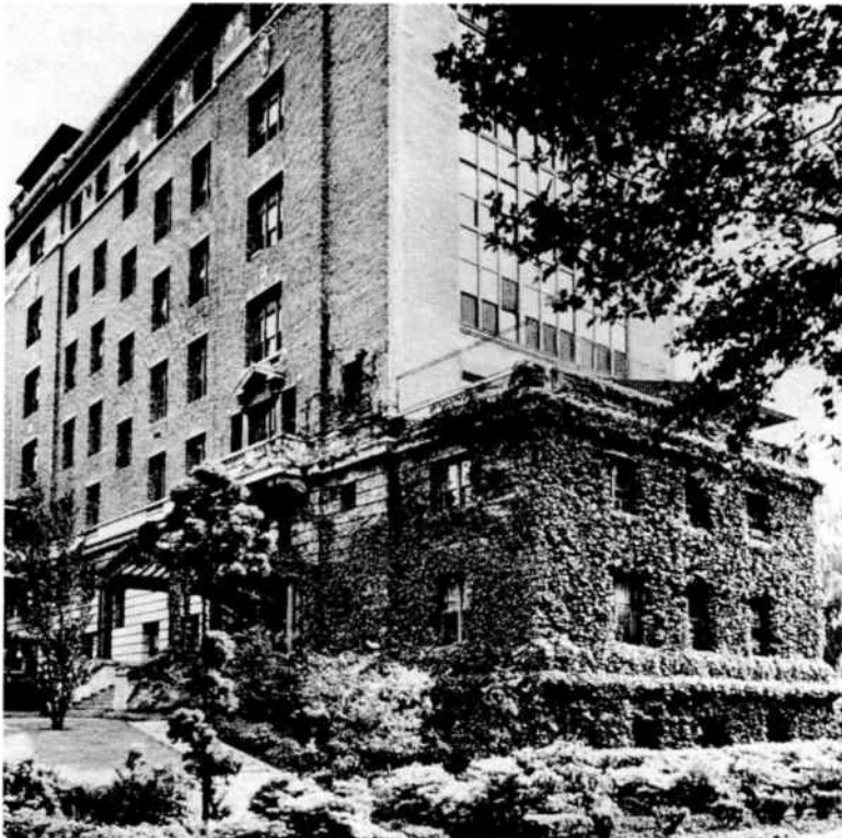
12 • The Hospital mellowed over the years as ivy began to cover its stark, utilitarian lines.
