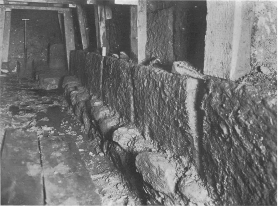
WALLSEND. FOUNDATION AND LOWEST COURSE OF THE WALL ; AT THE END OF THE TUNNEL IS SEEN THE JAMB OF THE FORT GATEWAY, OF ONE BUILD WITH THE WALL. (See p. 54). (Reprinted, by kind permission, from the Nor:umberland County History xiii. fig. 7).
