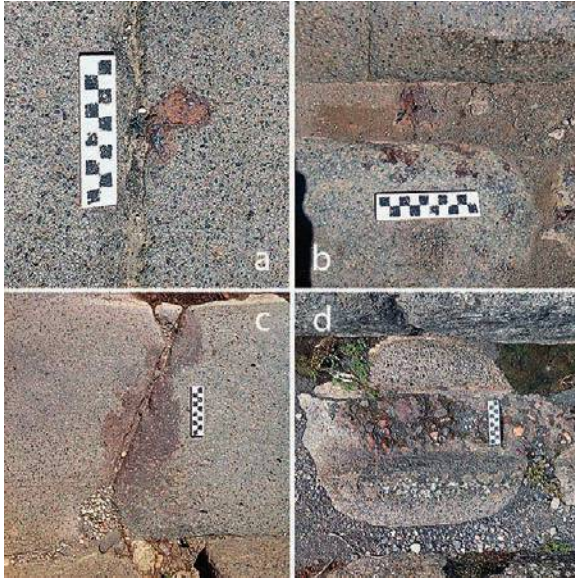
FIG. 15. Evidence of iron used to repair the streets of Pompeii: a, iron droplet; b, iron splatter and mass; c, iron staining; d, iron “slurry” filling rut.
