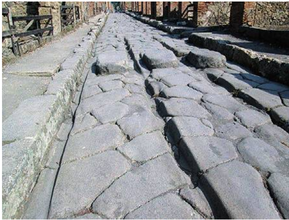
FIG. 4. Deep ruts on via Stabiana (PE_006) between vicolo di Balbo and via degli Augustali; view to north.
