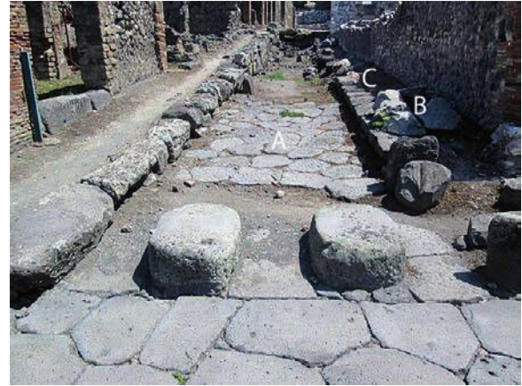
FIG. 16. Vicolo delle Conciapelle (PE_136) at via Stabiana (PE_097); view to east. Evidence for repaving in process: A, new paving; B, paving stone pile for reuse; C, paving stones recut into D-shaped curbstones.
