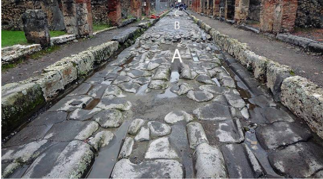
FIG. 6. Differential paving on via della Fortuna; view to west. Area of exceptionally deep ruts (A, PE_091) meets short section of repair (B, PE_090), followed by another deeply rutted section (C, PE_129).
