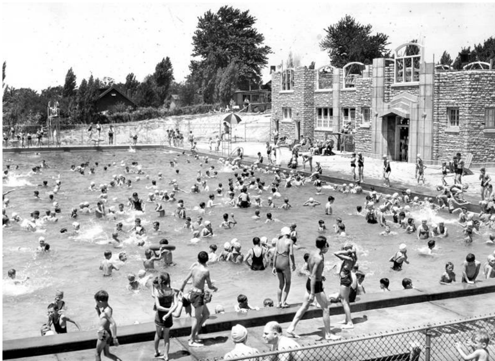
Figure 24 Maplewood Swimming Pool, St. Louis County, Mo., July 1938
