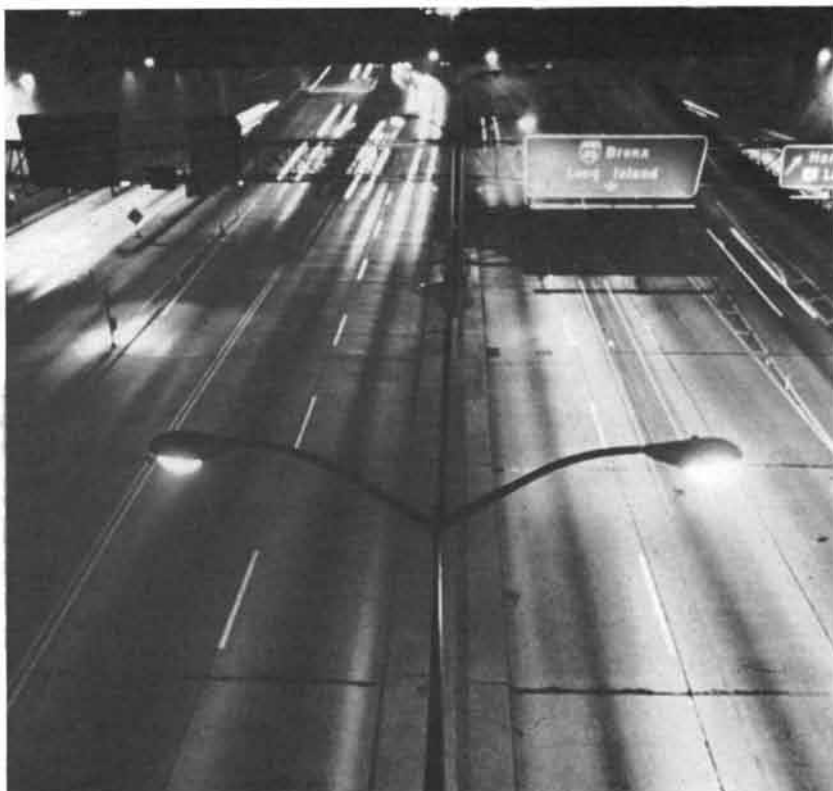
NIGHT LIGHTING of New York's George Washington Bridge shows contrast between the illumination from mercury and sodium high-intensity lamps. When the photograph was made, lamp standards over outbound lanes ( left ) contained 400-watt mercury-vapor lamps and those over inbound lanes ( right ) 400-watt sodium-vapor lamps. The illumination of the inbound lanes is two to three times brighter than the illumination of the outbound lanes.
