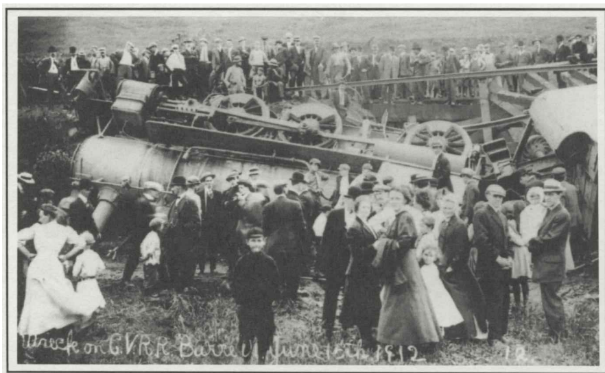
Fig. 12 —Although bridge failures continued to plague railroad travel early in this century, their number declined. This 1912 collapse of an old wooden bridge killed at least one man. (Courtesy Vermont Historical Society)
