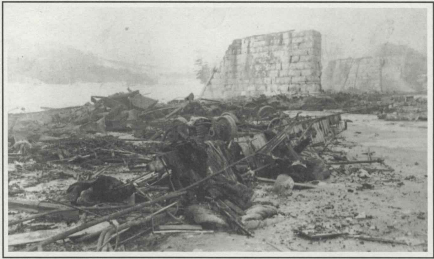
Fig. 7— What remained of the Woodstock bridge after the wreck of February 5, 1887. Engineers disagreed whether or not this constituted a bridge failure, because the accident resulted from a derailment and the bridge burned as a consequence. Yet, an adequately guarded bridge would probably have averted the tragedy. (Courtesy Vermont Historical Society)
