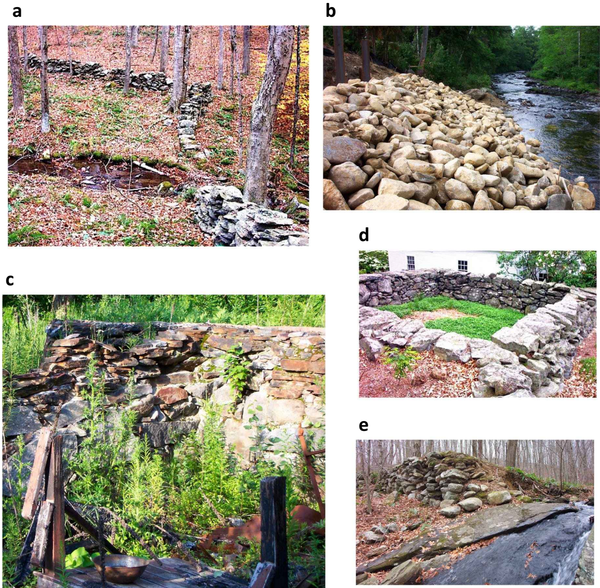
Fig. 15 Examples of all five families within the class Stone Wall. (a) Normal ( Subtype ) Single ( Type ) Freestanding ( Family ) wall in Storrs, Connecticut, has two faces. This is by far the most common type of wall in New England. (b) Armoring ( Type ) Flanking ( Family ) wall supports and prevents erosion of preexisting stream bank in interior Maine. Flanking walls have only one face. Note that stones support one another. (c) Small ( Type ) Supporting ( Family ) wall of cellar in southern
