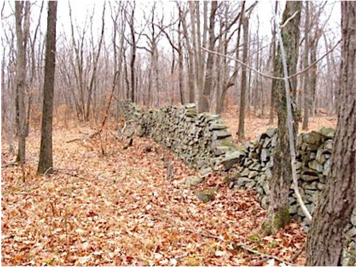
Fig. 1 This object is classified as a stone wall because it meets all five of the required defining criteria of: material (stone), granularity (population of stones), elongation (length/width >4), continuity (no breaks), and height (>knee-high or stone-on-stone). Taxonomically, it is the Fitted Variant , of the Panel
