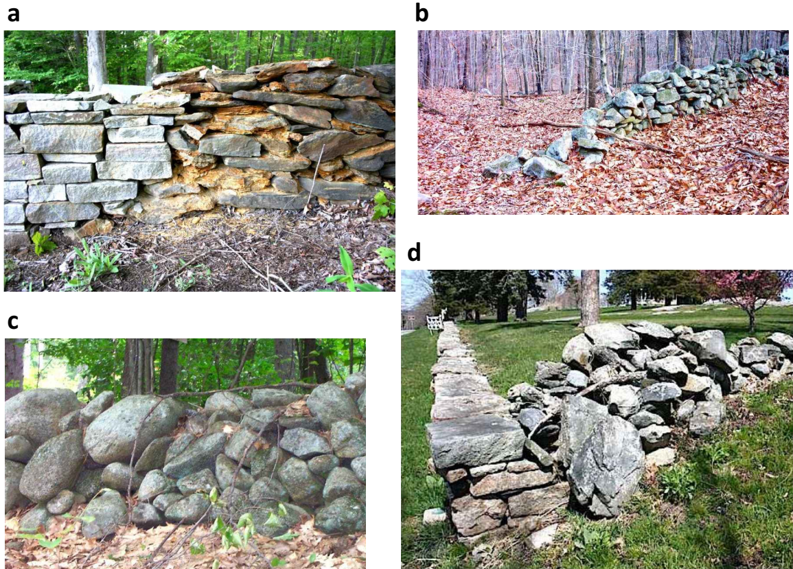
Fig. 8 Examples of contrasting terminations (ends of walls) and contacts (ends of wall segments). (a) Segment of laid double wall of quarried granite slabs was built against a disintegrating segment of single wall dominated by quarried (pyrrhotite-bearing) schist. By definition, this one wall has two abutting segments with a non-vertical contact. (b) Unbuilt tip of final segment of single wall is a termination. (c) Wall in
