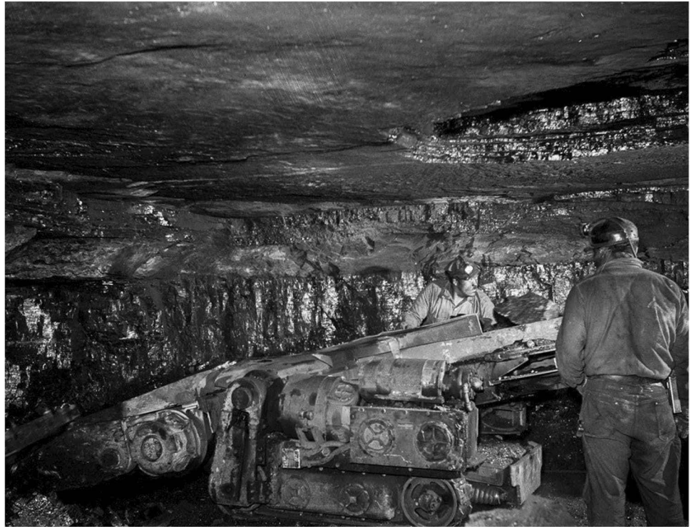
Fig. 2 Two miners loading coal beneath unsupported roof prior to the Mine Act. Note where a portion of the roof has already fallen out. Such photographs were quite common in that era, further indicating that the practice of working beneath unsupported roof was widespread (source: US Bureau of Mines)
